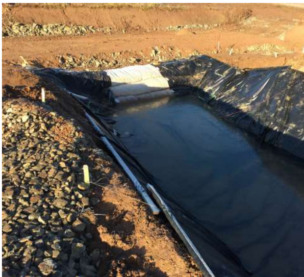
Different test scenarios were undertaken to proof dam stability and safety.
