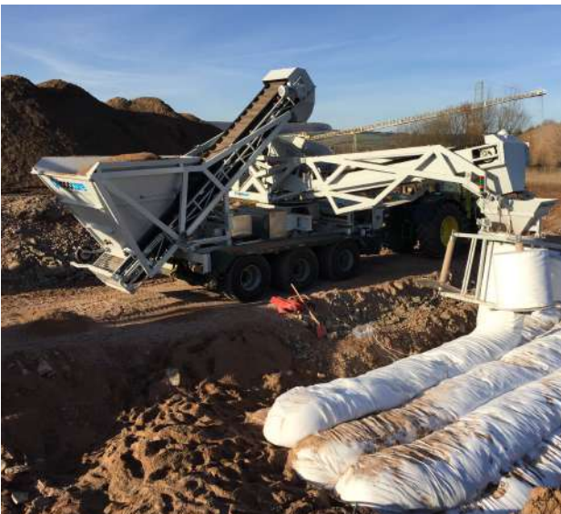
The boom is fully variable to facilitate different dam designs.
