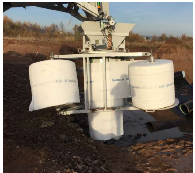
The tubes are produced directly on site using our unique helix system.
